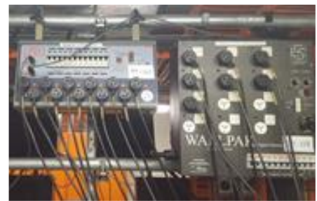
Piggyback plugs used with lighting dimmers
